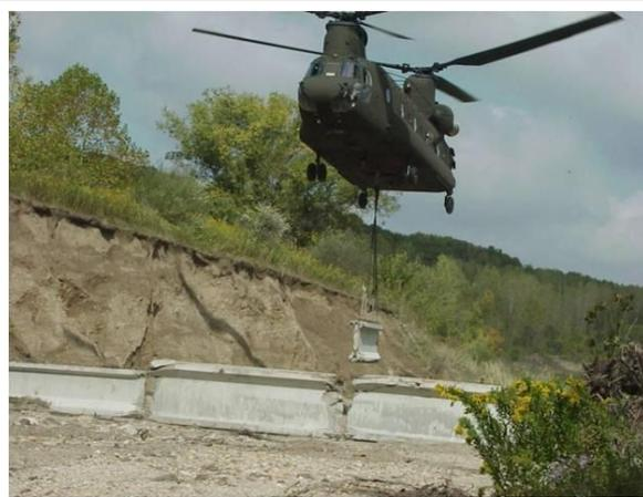
Training activities were incorporated into the restoration construction; here, helicopter training is used to move concrete beams into place.
