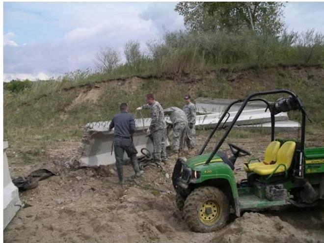
Riffle construction was undertaken at MTC to correct legacy erosion issues and achieve shared interagency goals for creek restoration.
